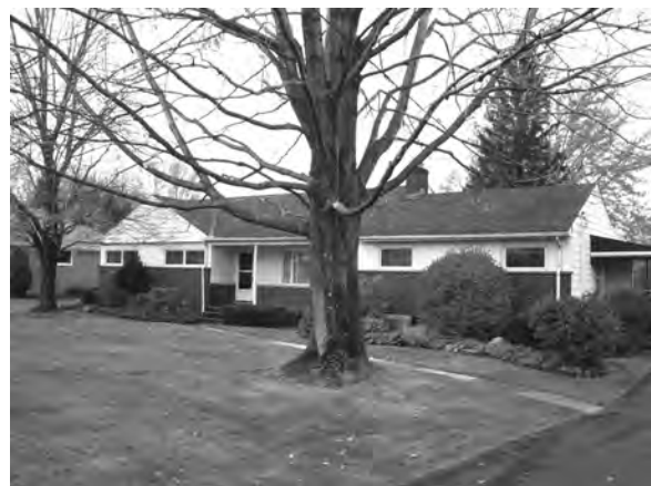
Renovation work on this home in Richmond Heights has begun. When completed this will be the home for 4 tenants.
